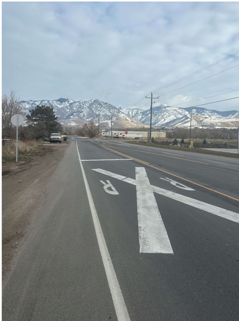
Figure 1 – 11600 South looking east.
